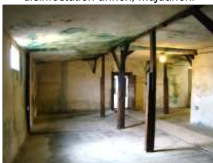
Inside walls of fumigation chamber, Building #41, Majdanek.
